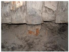
supports installed under the floor joists of the west side of the cabin, from the front door to the end of the bathroom. After that, other restoration such as replacing the base course on the west side of the cabin can be done.
